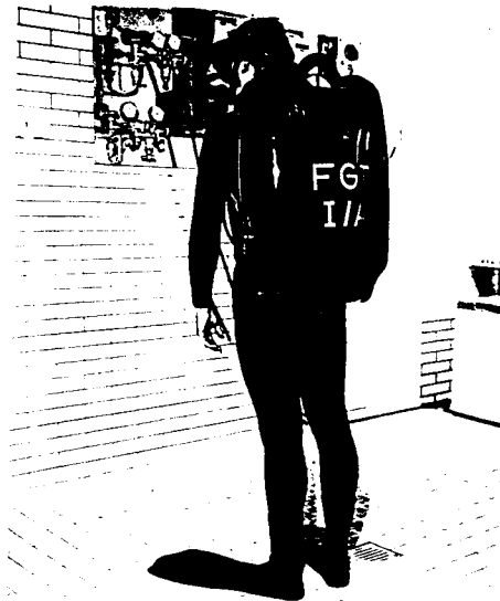
Fig.1 Mixed-gas swim-diving apparatus FGT I/A
